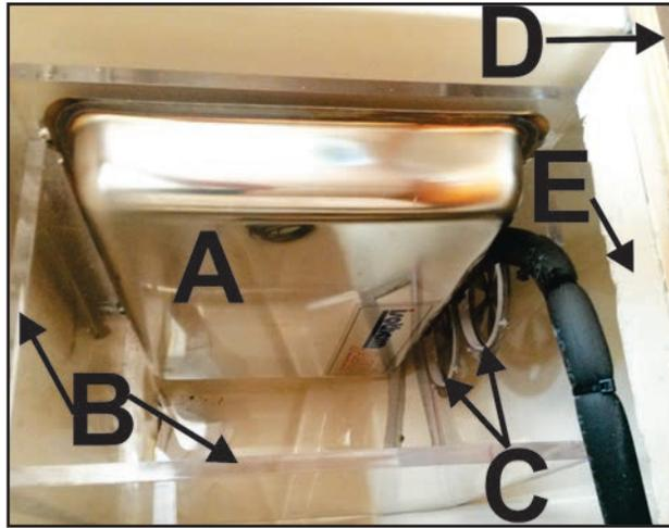
Figure 4: This image is looking into an open, insulated box where the holding plate "A" is mounted in the Plexiglas box, "B". "C" is the adjustable vents that are used to regulate the amount of cold that flows out of the freezer into the refrigerator space. "D" is the seal all around the opening for the lift out, and "E" is the foam insulation on the inside of the top.
